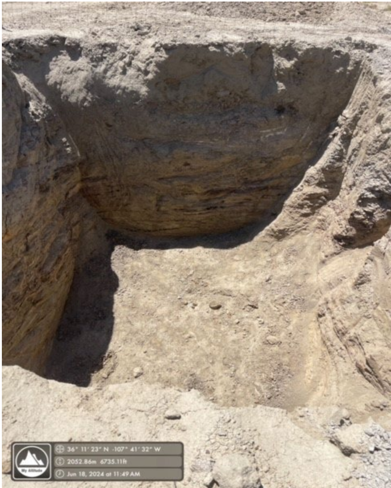
Photo 4: BGT Berm South Wall
