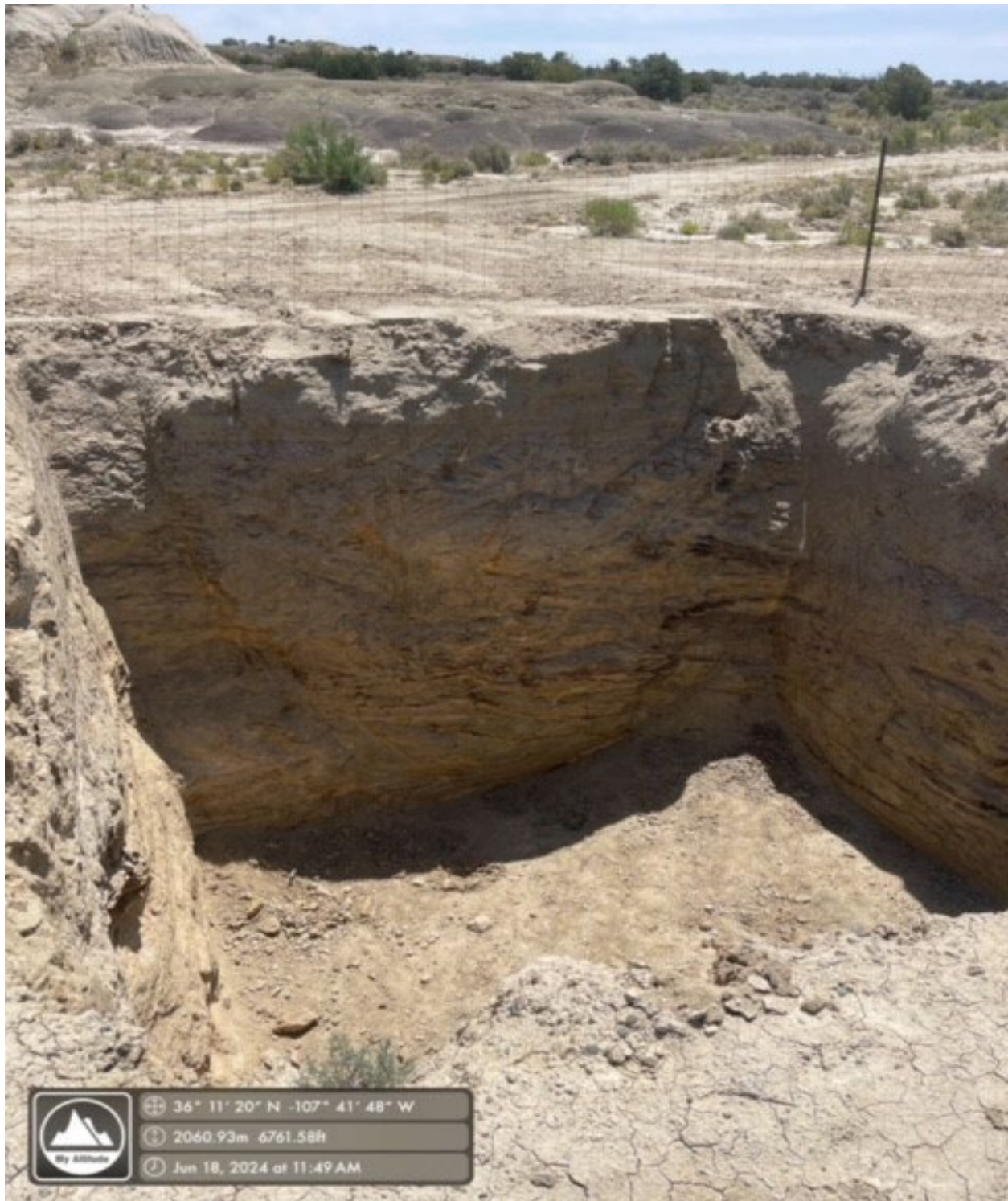
Photo 2: BGT Berm East Wall
