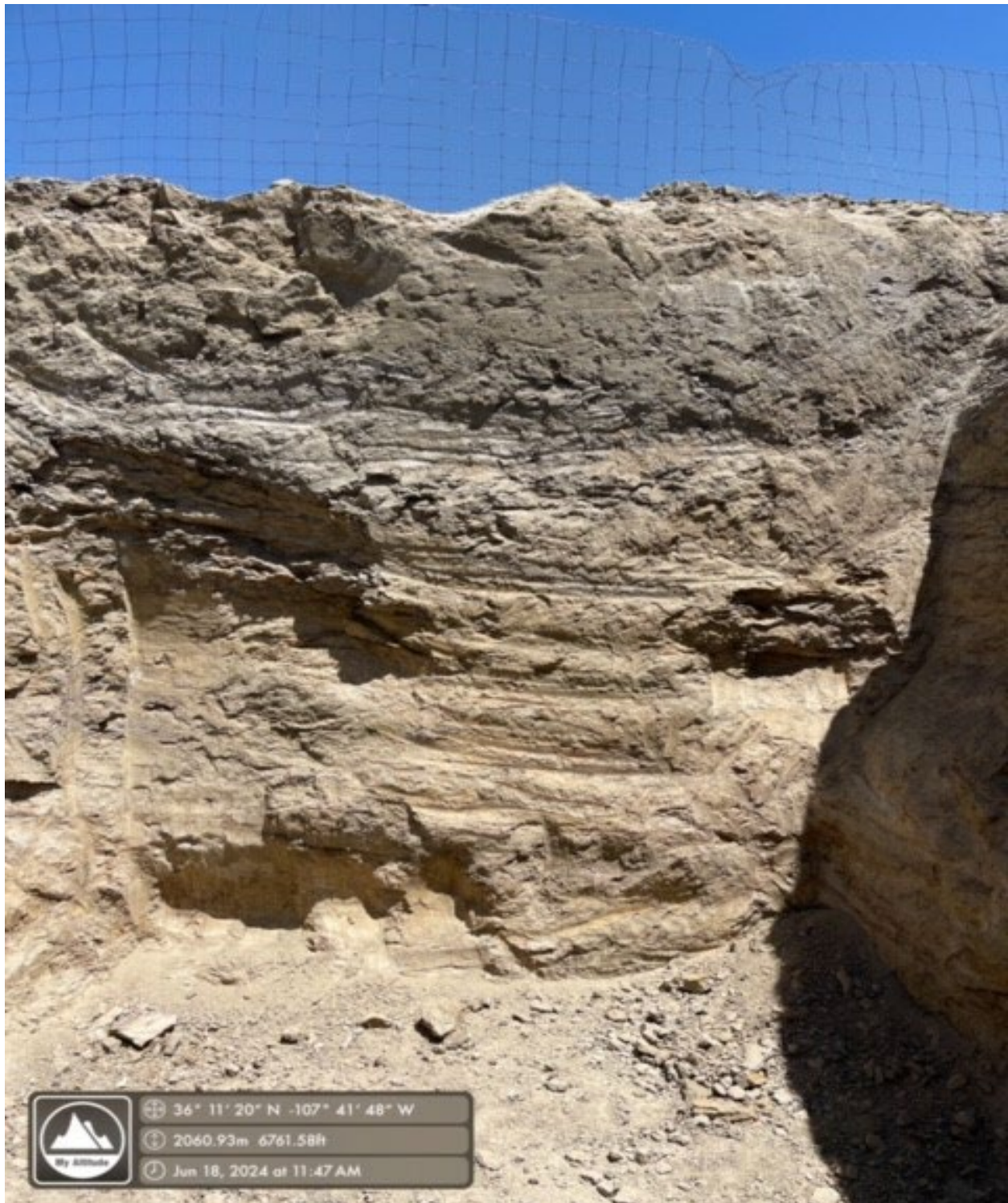
Photo 3: BGT Berm North Wall
