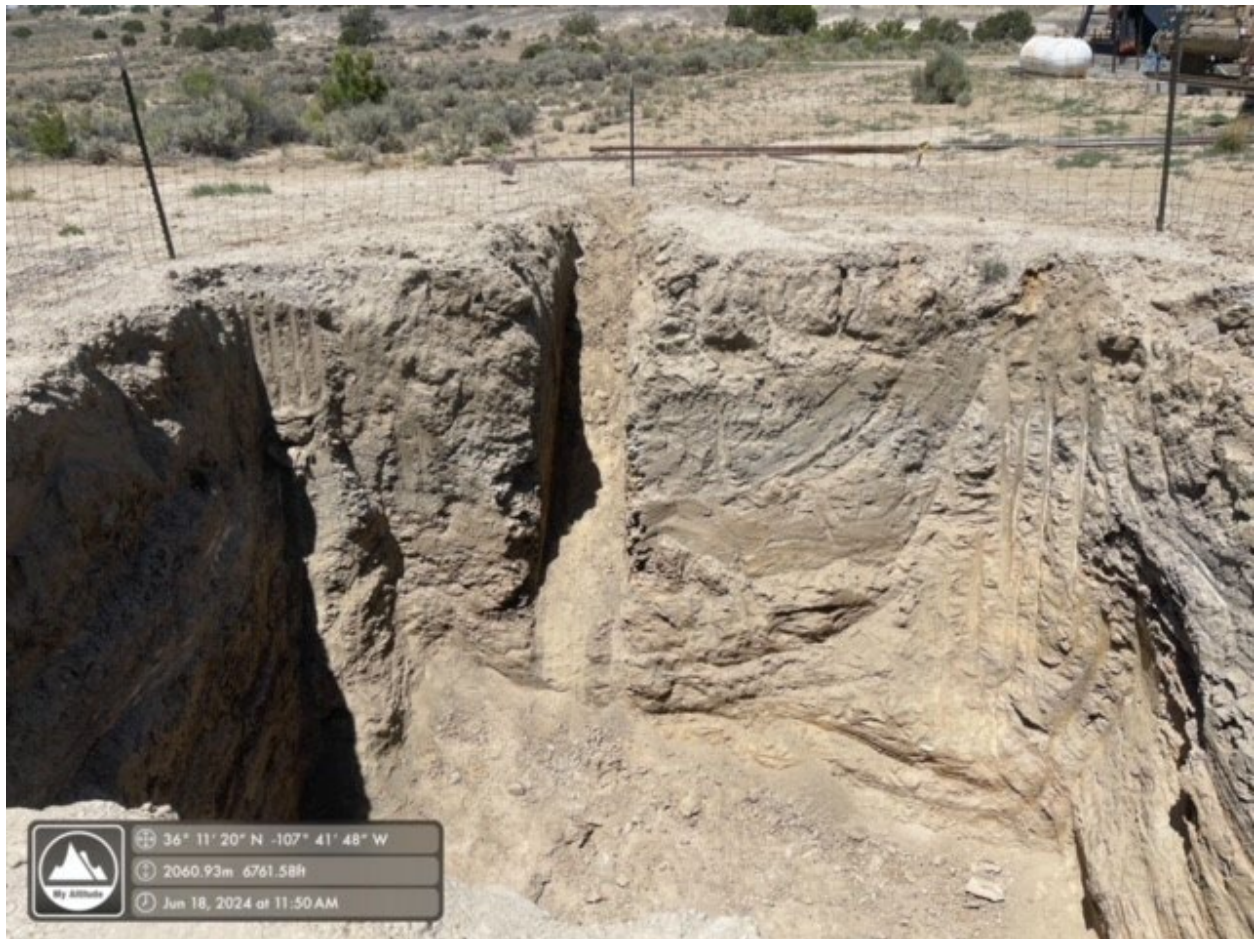
Photo 5: BGT Berm West Wall
