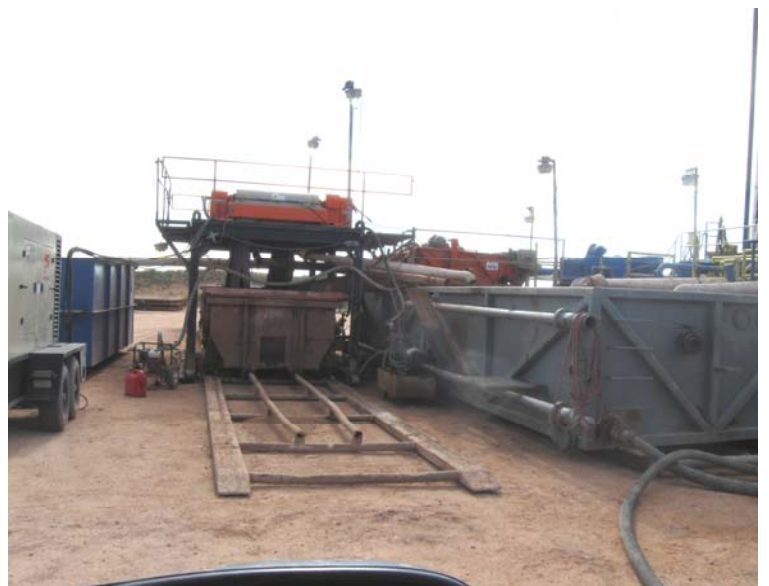
Above: Centrifugal Closed Loop System
