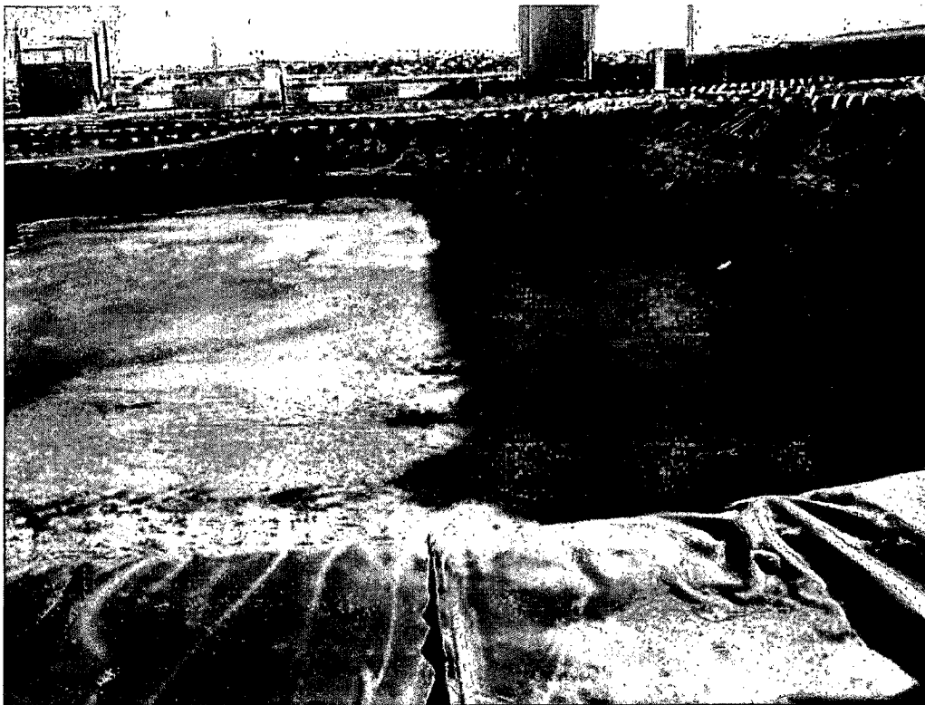
Photo 2: Mud exposed in pit after removing most of the fluid (looking south).
