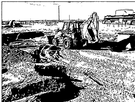
backfilling the site with caliche, facing northwest 11/30/2012
