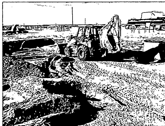
backfilling the site with caliche, facing northwest 11/30/2012
