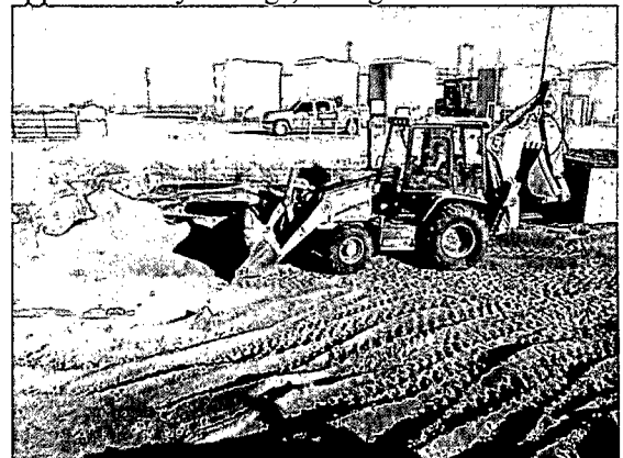
padding above the liner with blow sand, facing north 11/30/2012
