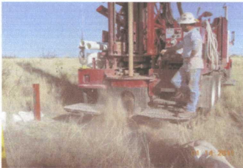
drilling MW-1R (facing east)
