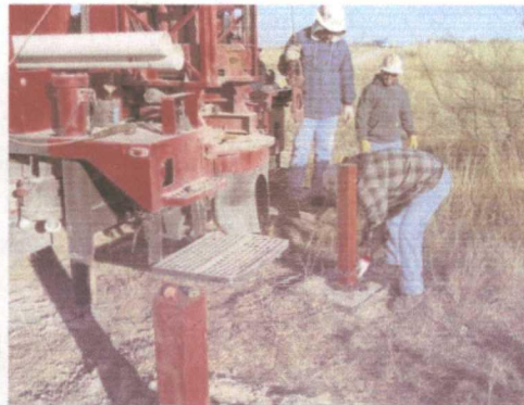
preparing to remove MW-1, facing north 1/21/2011
