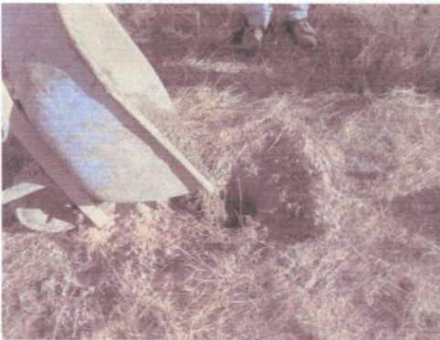
plugging MW-1 with concrete/bentonite slurry 1/21/2011
