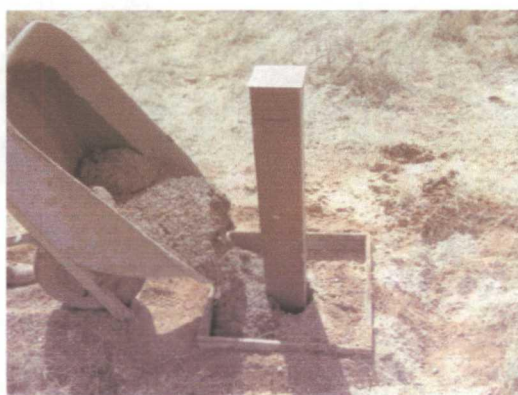
Pouring the concrete for the base
