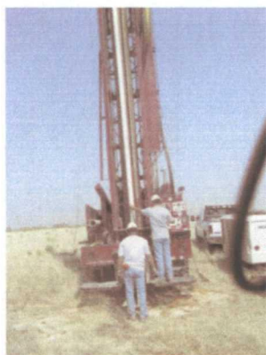
Inserting the casing into the hole
