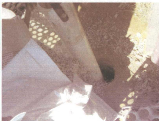
Adding the bentonite seal
