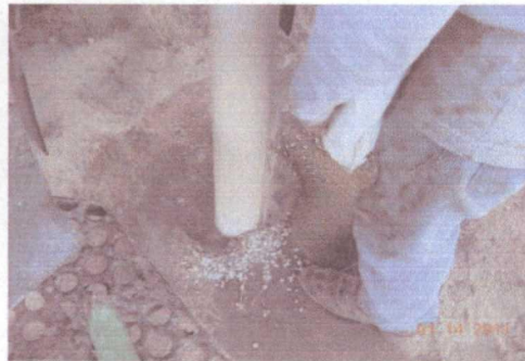
sealing the well in with bentonite (facing south)
