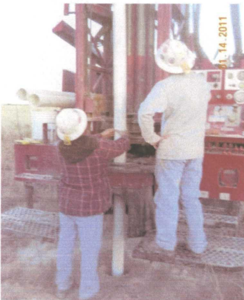
setting the casing (facing east)
