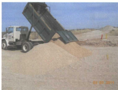
importing base coarse for lease road construction
