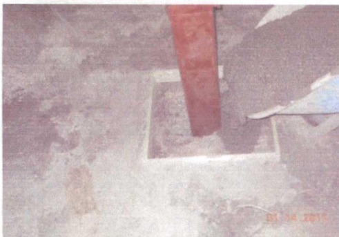
concreting the well in (facing south)
