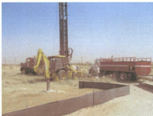
Drilling RW-2 with mud rotary (facing south-east)
