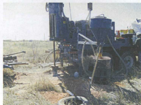
Photograph 7. Air rotary drilling Chinle Formation at MP-1.
