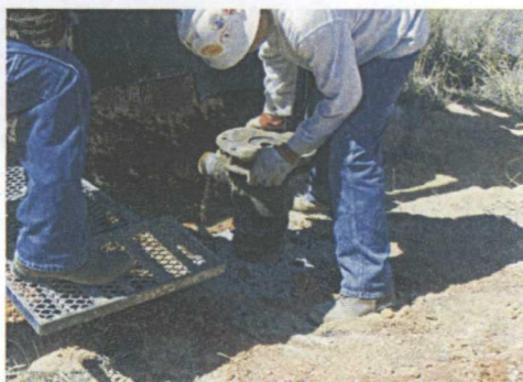
Photograph 5. Converting from HSA drilling to air rotary at MP-1 (also typical of other boring locations).
