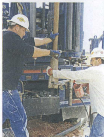
Photograph 6. Converting to air rotary drilling at MP-1 (also typical of other boring locations).
