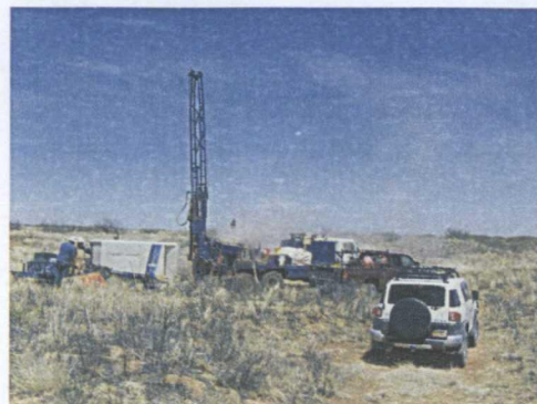
Photograph 19. Rodgers set up on MP-4 with CME-75 combination HSA and air rotary drill rig and related equipment.
