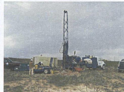
Photograph 20. Rodgers set up on MP-5 with CME-75 combination HSA and air rotary drill rig and related equipment.
