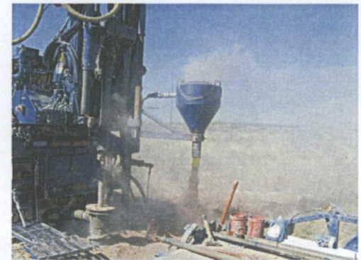
Photograph 12. Air rotary drilling dry Chinle Formation at MP-2.
