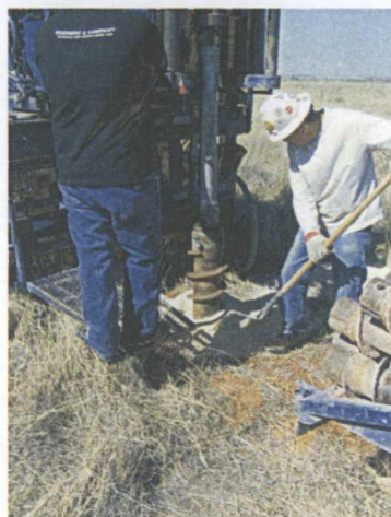
Photograph 2. HSA drilling MP-1.
