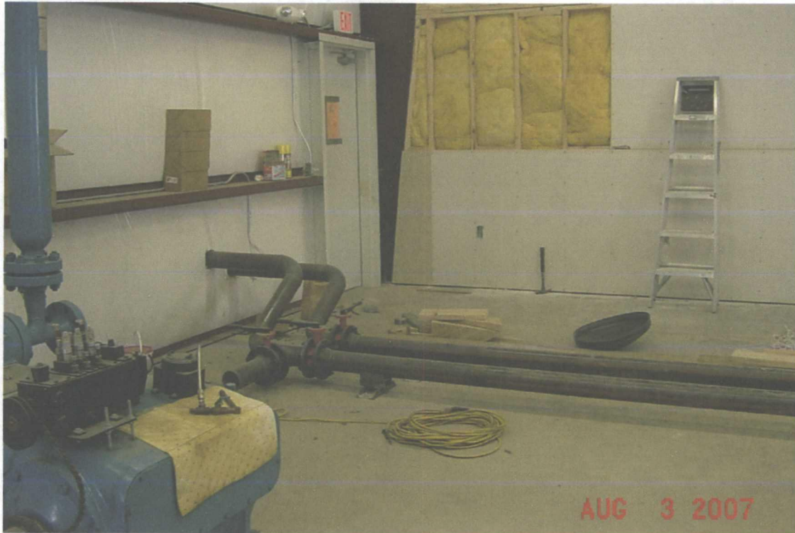
Picture 7. In-flow from raw water storage and outflow to brine storage tanks
