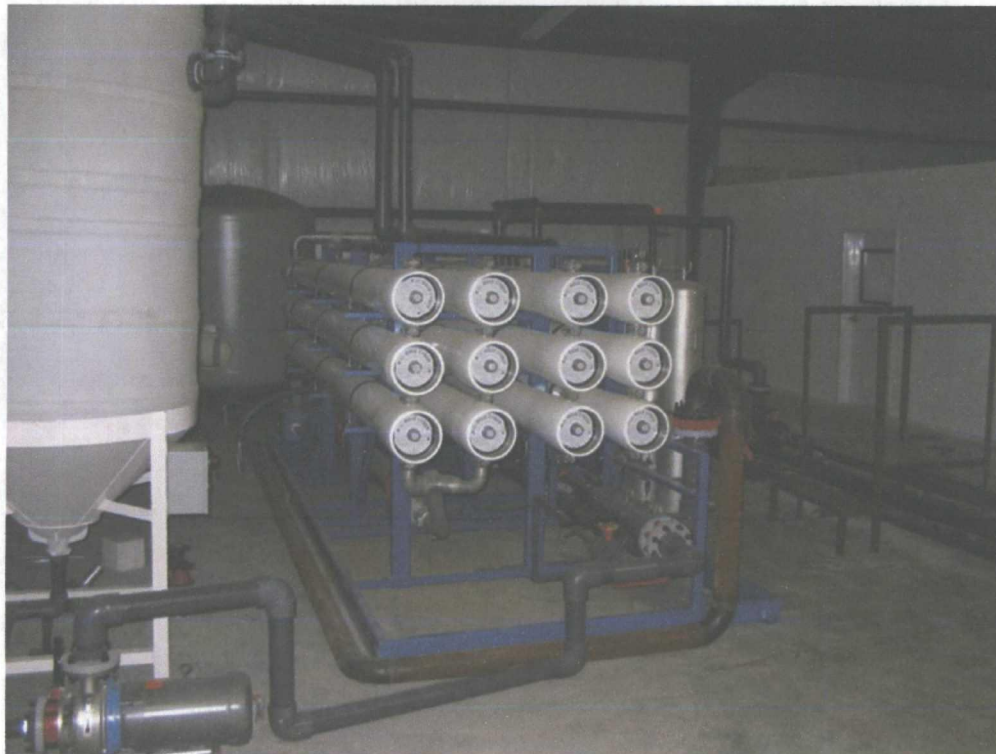
Picture 22. RO apparatus (large tank to the left allows the filter system to be cleaned in place)
