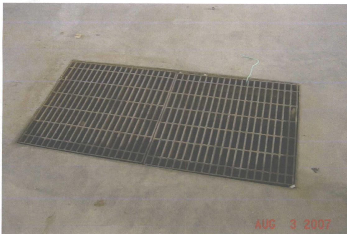
Picture 4. Drain under intake connected to sump tank
