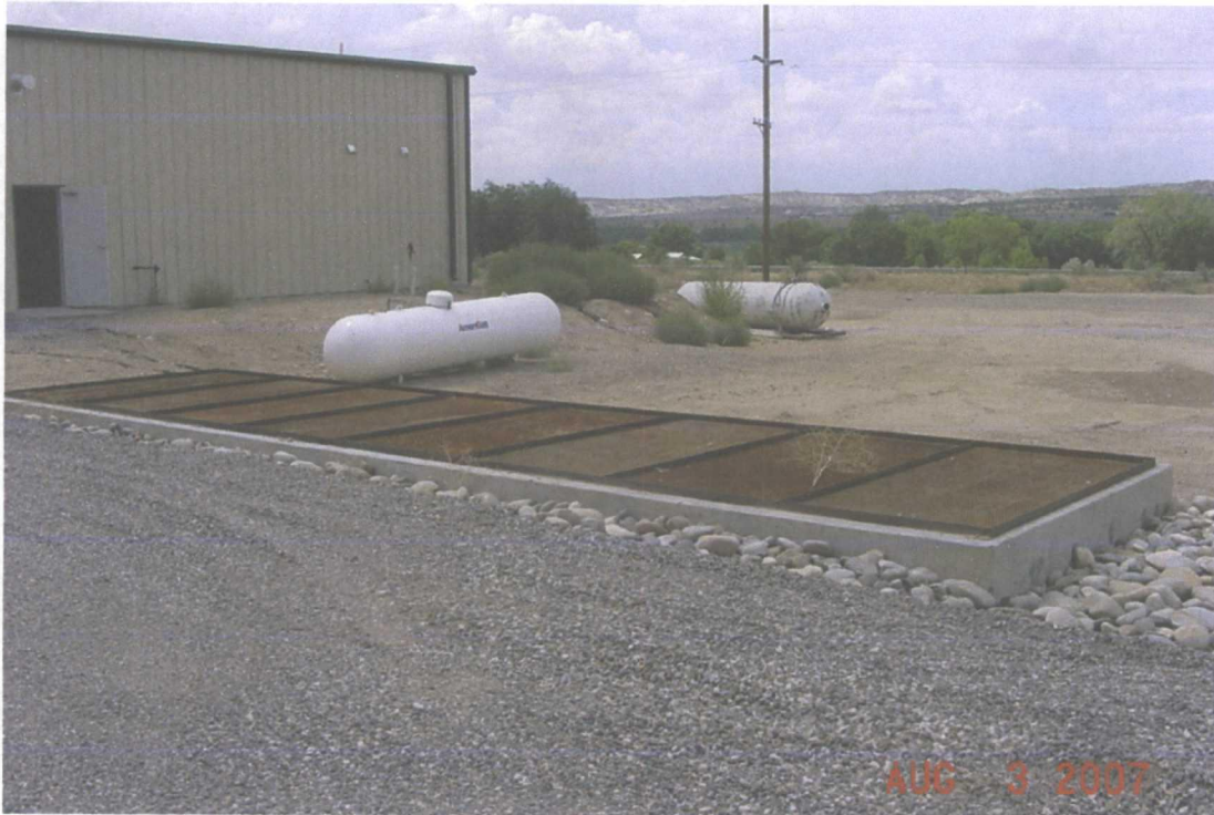
Picture 5. Concrete Sump Tank 350 bbl connected to floor drains
