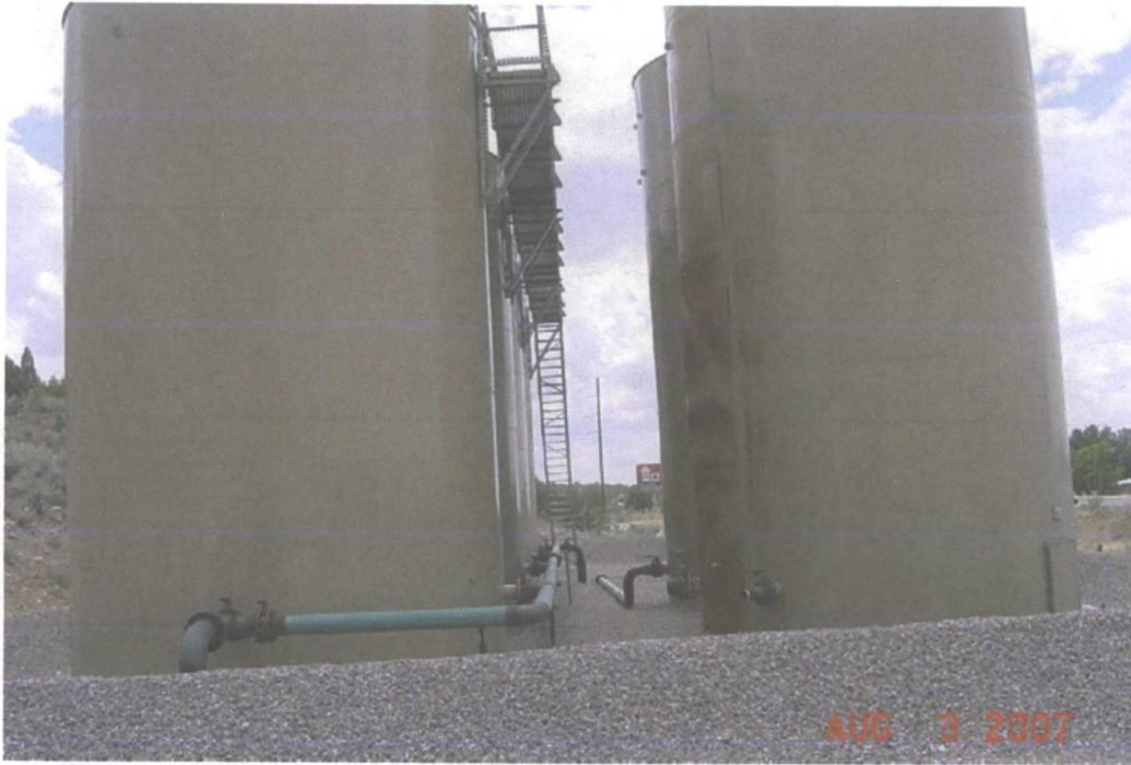
Picture 1. Raw water storage tanks
