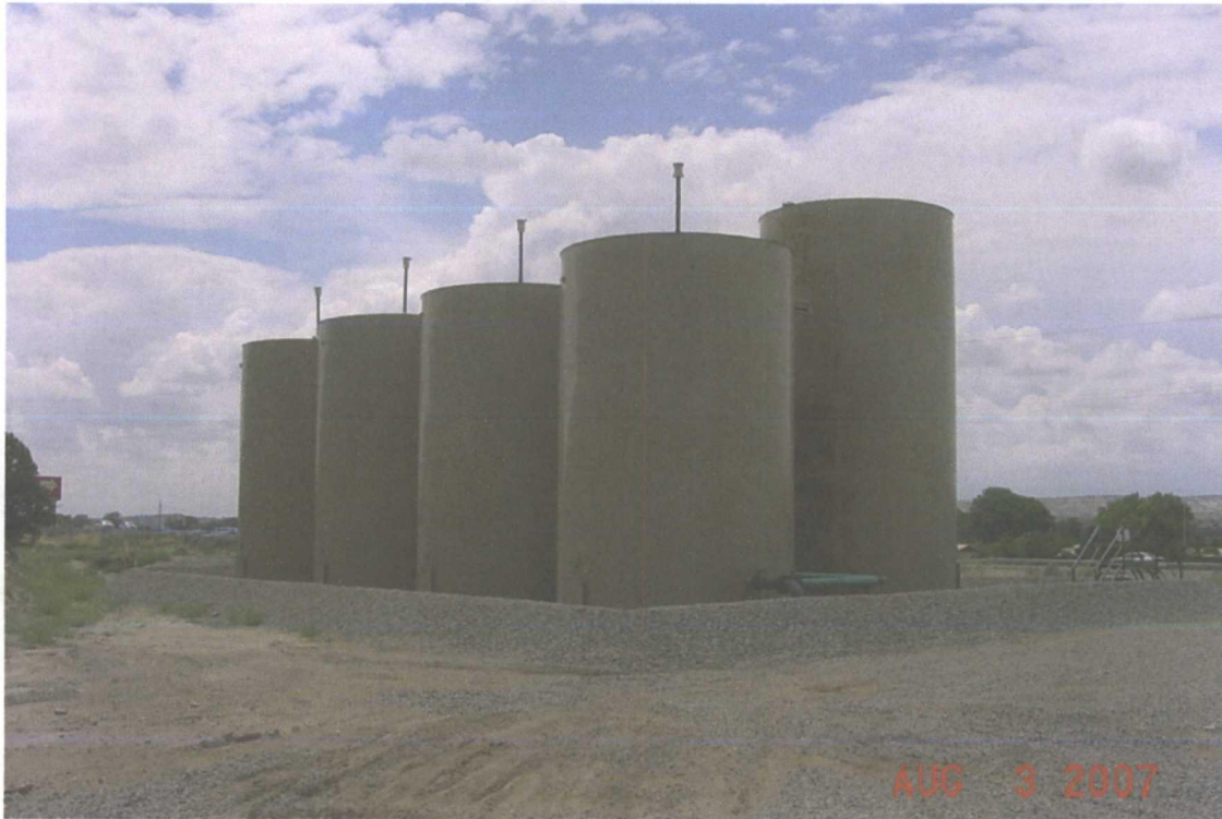
Picture 13. Raw (left) and Brine (right) water storage tanks
