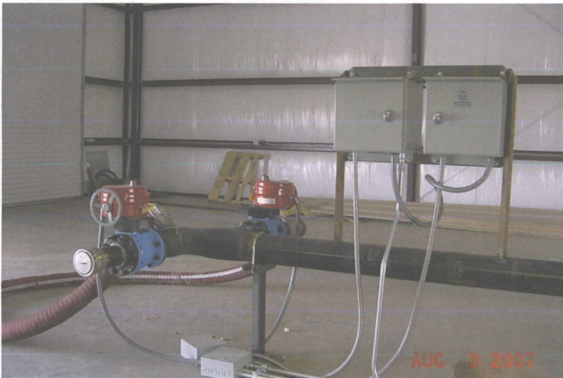
Picture 12. Pin box and actuator for water delivery
