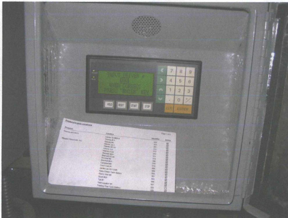
Picture 20. Driver & Location Key Box (must activate before off-loading)
