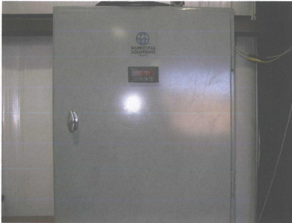
Picture 19. Settling Tank Control/Monitoring Panel (visible to drivers)
