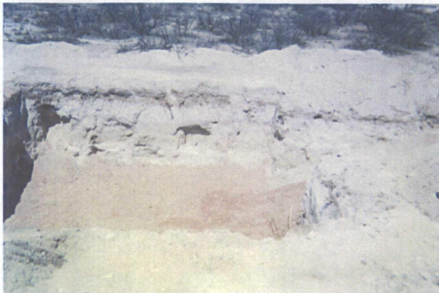
Clay liner installed
