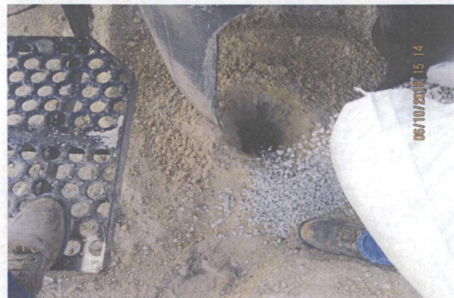
Soil bore # 1 plugged with bentonite
