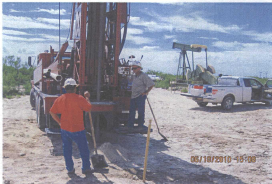
Drilling soil bore # 1
