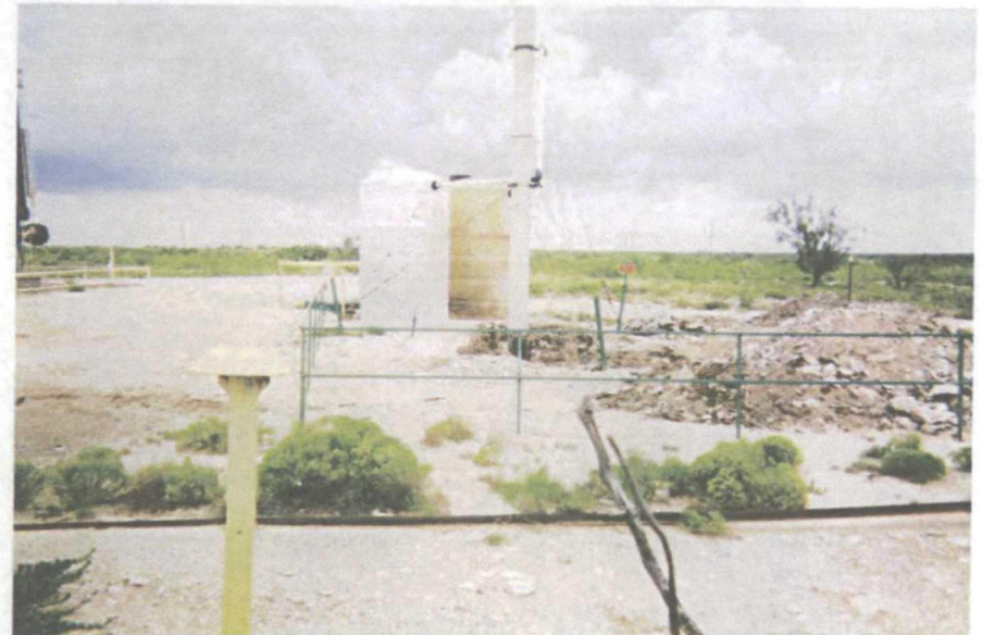
junction boxes removed, facing north
