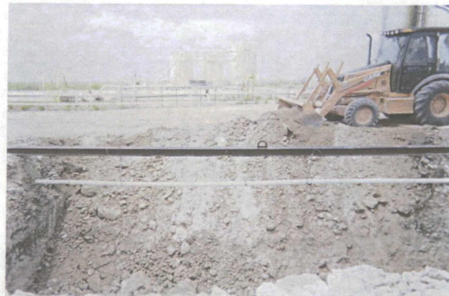
backfilling excavation, facing west
