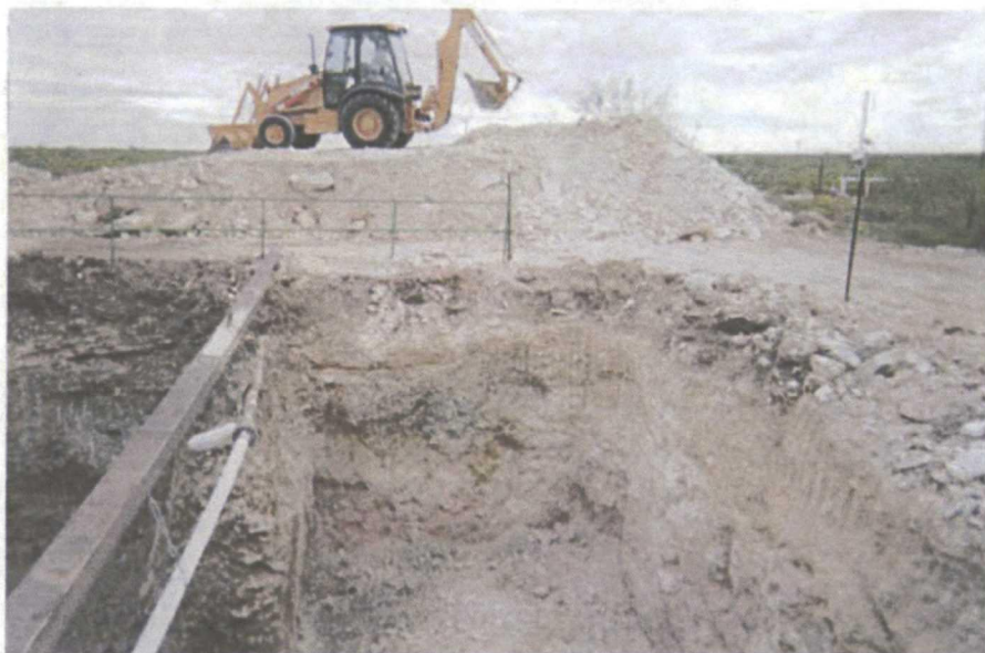
excavation, facing east
