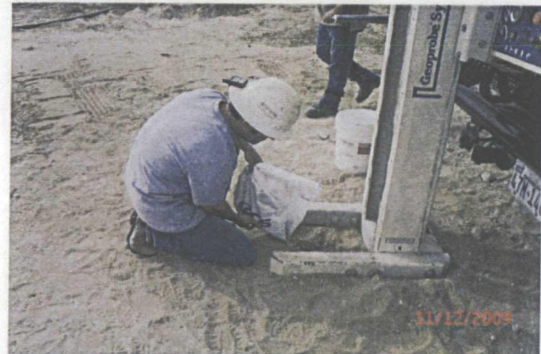
plugging SB #1 with bentonite
