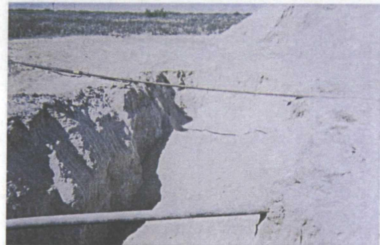
backfilling the final excavation up to 5 ft BGS, facing east
