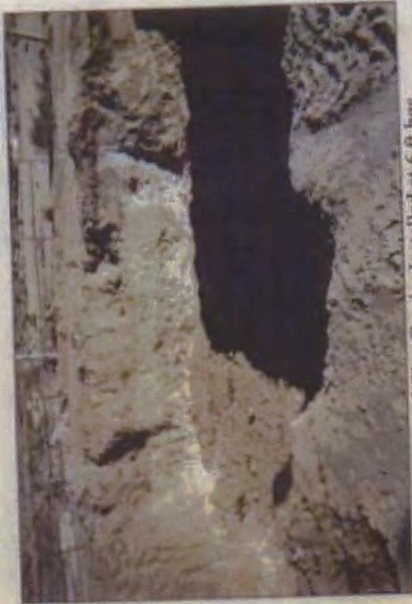
Compacted Clay Barrier Installed at 6 ft bgs
