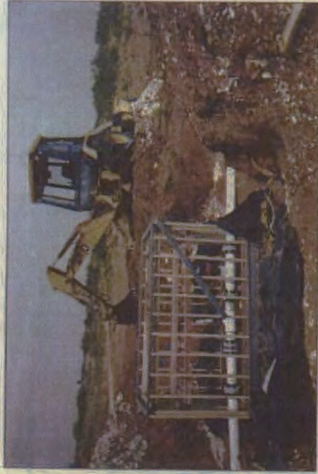
Construction of New Junction Box 50 ft East
