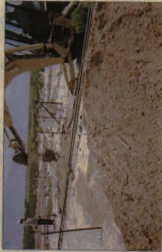
backfilling old box location with clean fill
