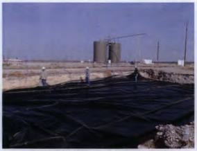
Installing the 20-mil, reinforced liner at approximately 4.5 ft bgs, facing northwest 3/27/2013
