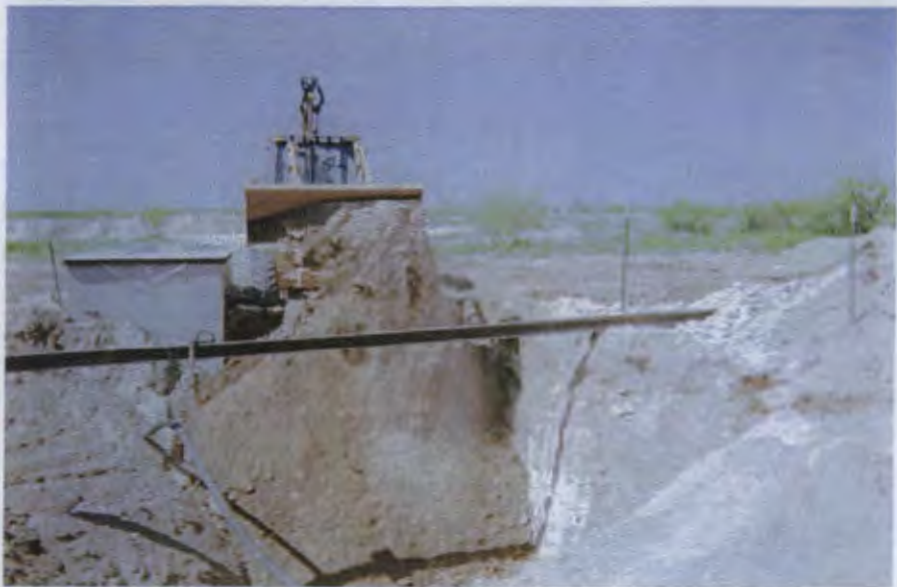
backfilling excavation up to 6 ft BGS
