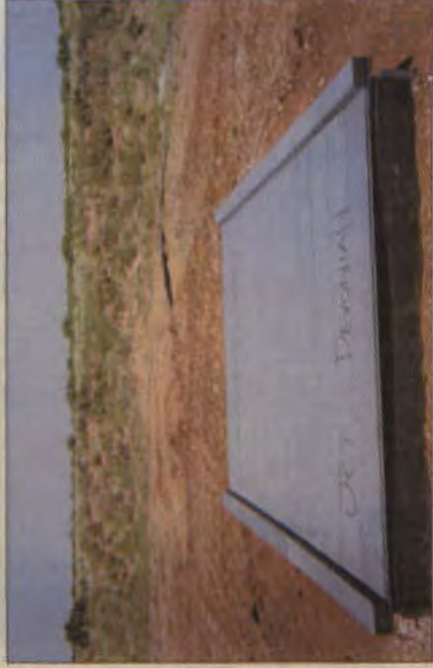
completed new watertight junction box 167 ft north
