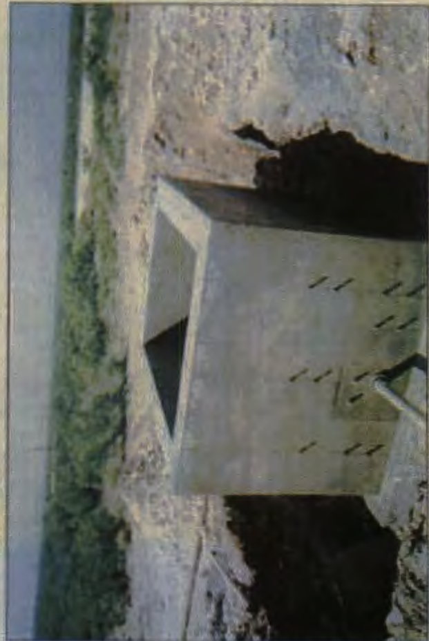
construction of new junction box 20 ft southwest of former
