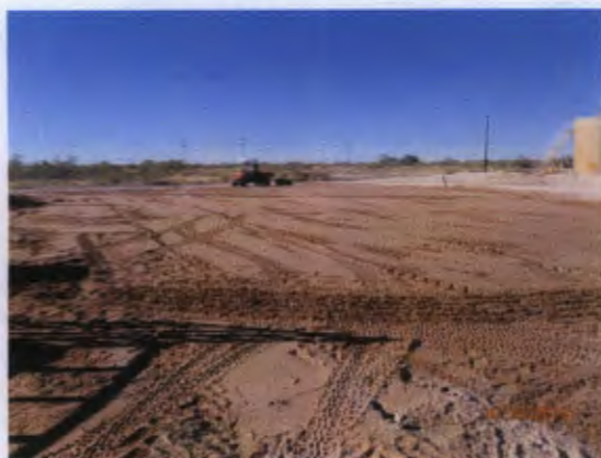
Discing the backfilled site, facing southwest
