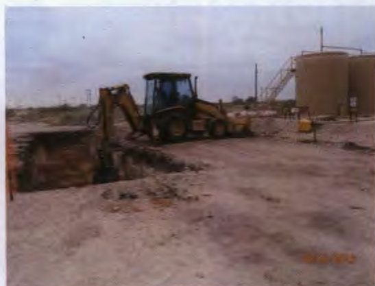
Padding the west excavation with blow sand, facing southwest 10/16/2013
