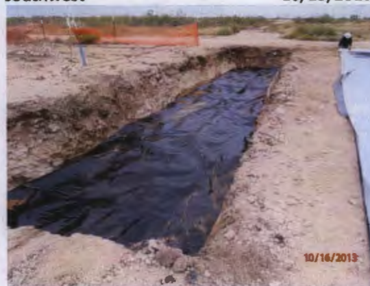
20-mil, reinforced liner installed, facing southeast 10/16/2013
