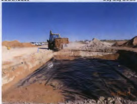
Padding the 20-mil, reinforced liner with blow sand, facing north
