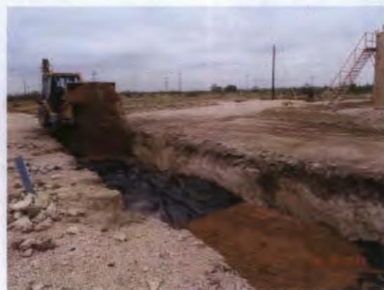
Padding the liner with blow sand, facing southwest 10/16/2013
