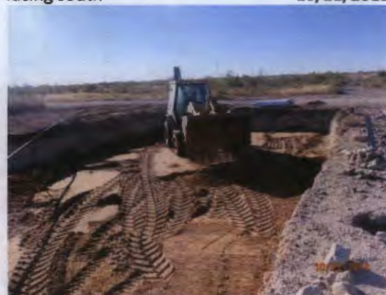
Padding the excavation with blow sand, facing southeast
