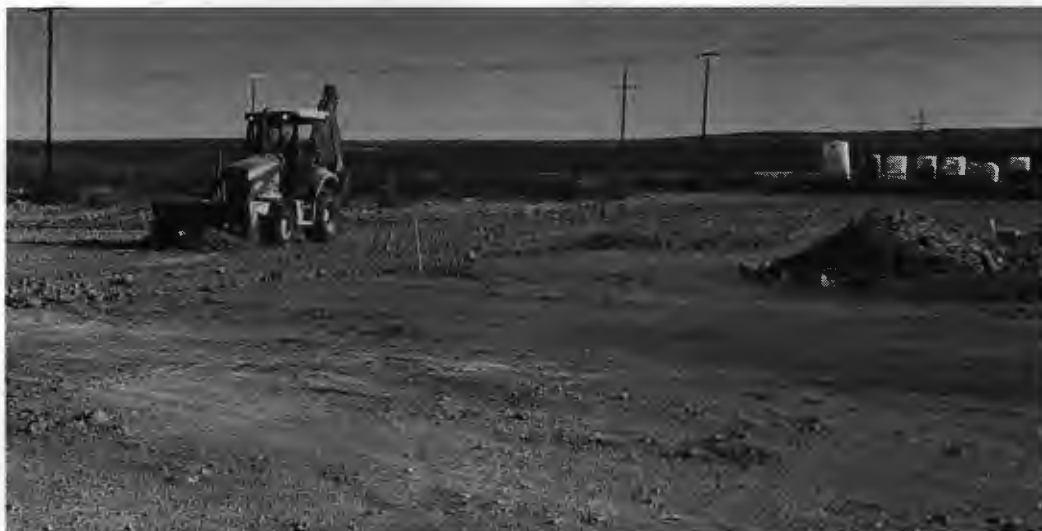
Figure 2: Grading of former containment berms. The former berms were either thin spread on location or placed around location to reinforce existing berms (Figure 3).
