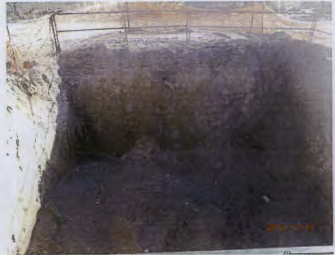
Installed 6" sand pad at base of excavation, facing south
