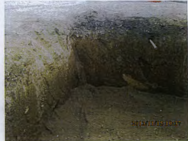
Installed 6" pad above liner, facing northeast
