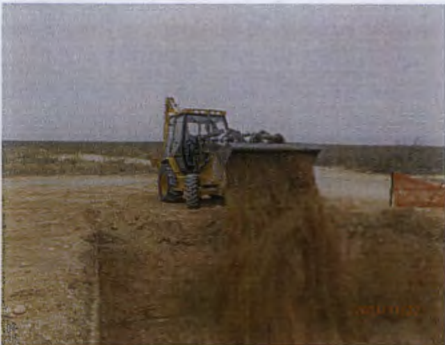
Backfilling excavation, facing southeast
