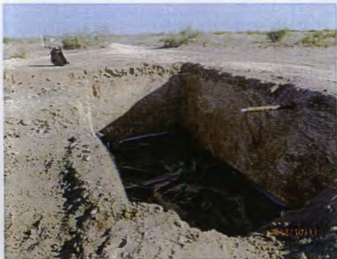
Installed 30'x15' 20-mil liner at 11'ft bgs, facing northeast 10.11.13
