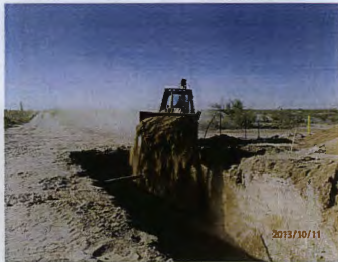
Installing 6' pad above liner, facing southwest 10.11.13
