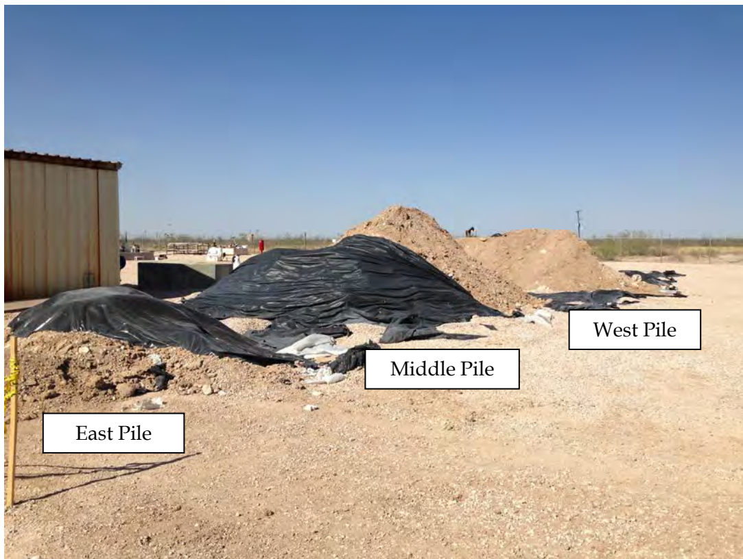
Excavated Material April 29, 2014
