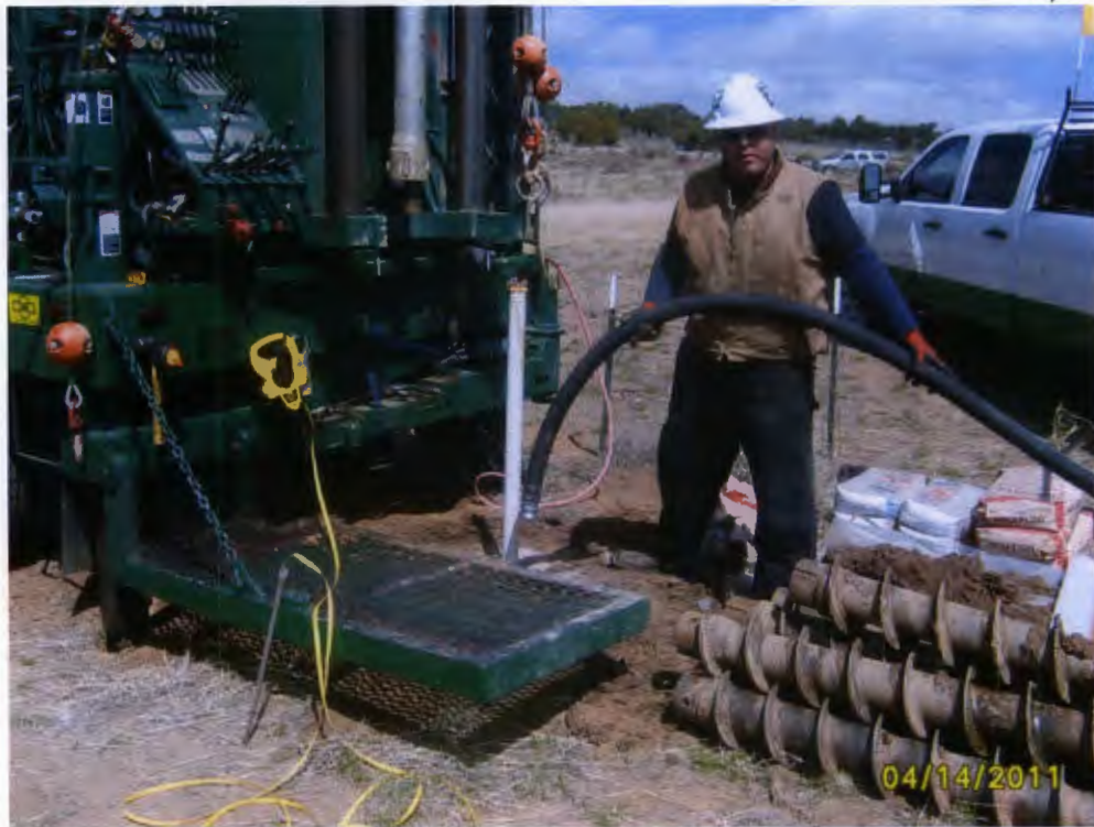
7. April 14, 2011: Facing N, hydrating bentonite seal of MPE-6.
