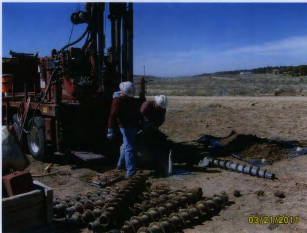
2. March 21, 2011: Facing SW, pouring cement grout at MPE-5.
