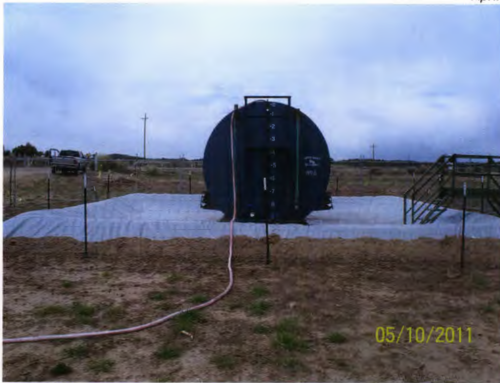
11. May 10, 2011: Facing N, 210-bbl tank used to collect produced water and crude oil.
