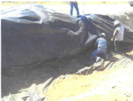
installing a 20-mil, reinforced liner
