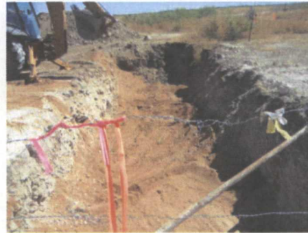
50x17-ft excavation padded with 6" blow sand, facing south
