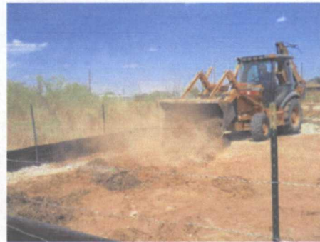
spreading imported blow sand blended with peanut hay, facing east
