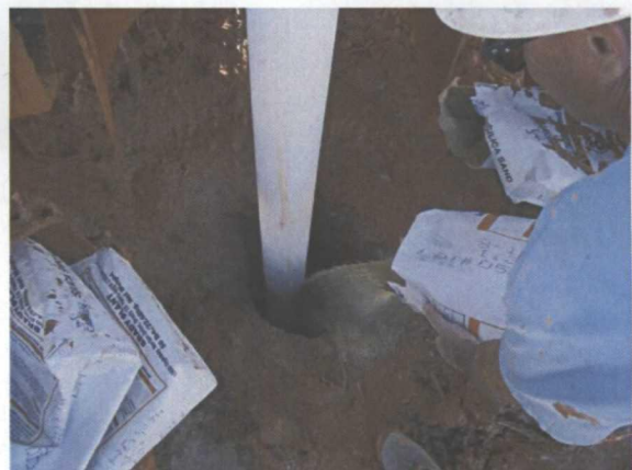
Inserting silica sand pack
