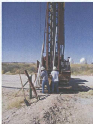
Inserting the casing, facing north
