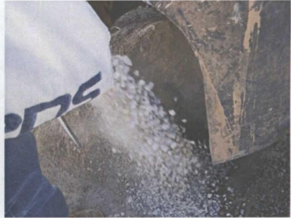
Plugging the soil bore with bentonite
