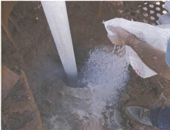
Adding the bentonite seal
