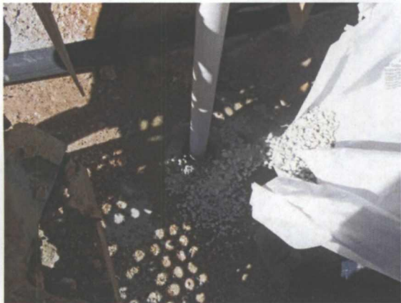
Adding the bentonite seal
