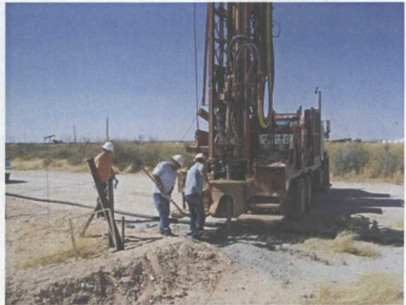
Drilling MW-2
