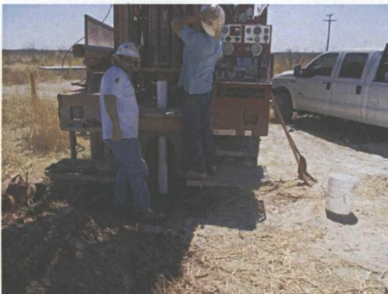
Inserting the casing into the well
