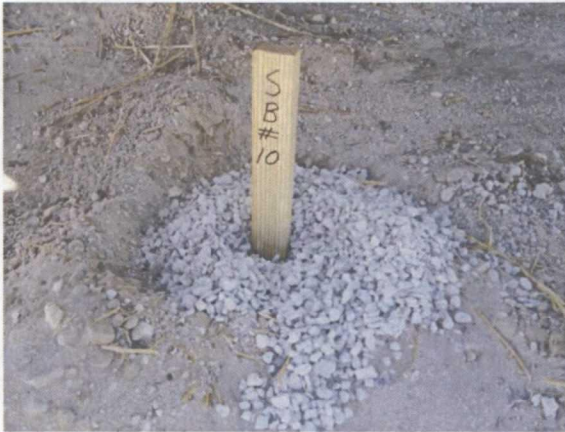
Completed soil bores
