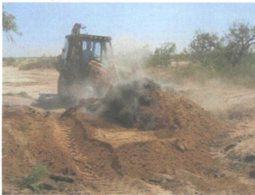
blending the imported soil with peanut hay
