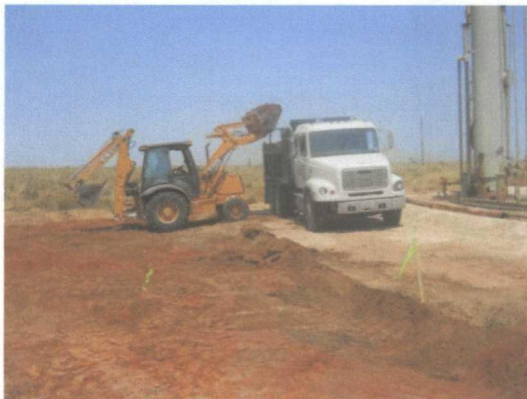
scraping the site to a depth of 6 inches and hauling off soil, facing west
