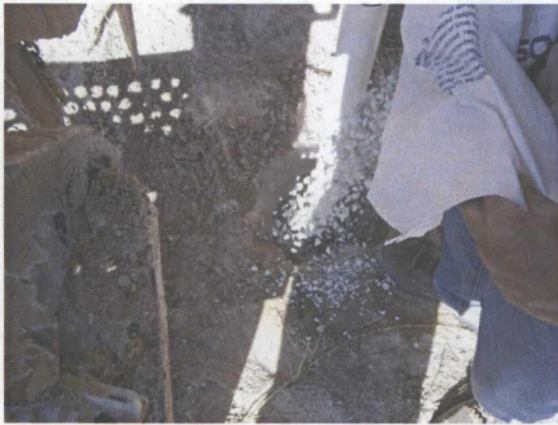
Adding the bentonite seal
