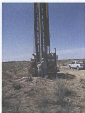
Inserting the casing into the well
