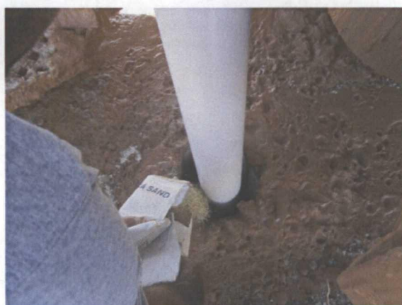
Inserted silica sand pack
