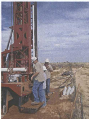
Inserting the casing
