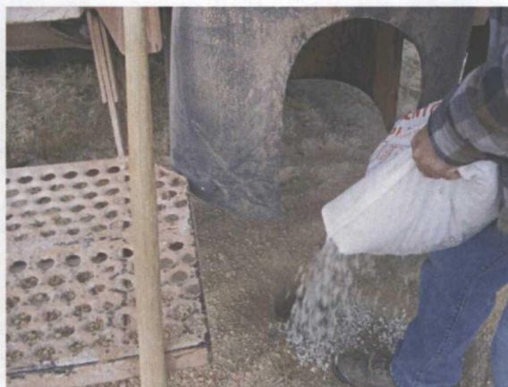
Plugging the soil bore with bentonite
