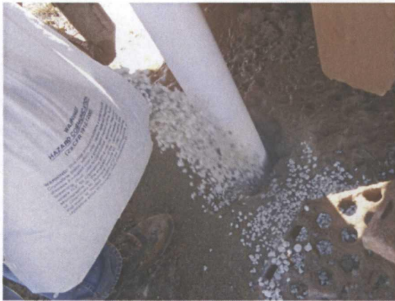
Adding the bentonite seal
