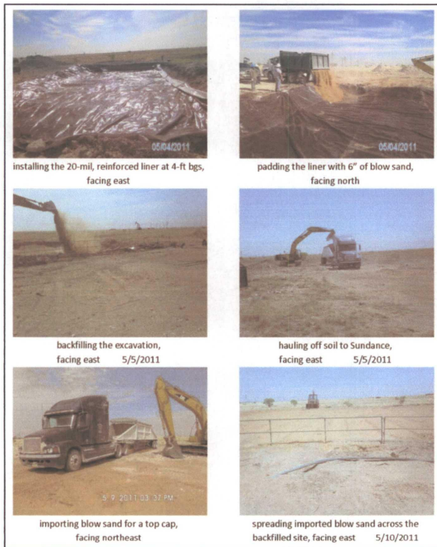
Figure 2c – Photo-chronology of double-liner installation and soil restoration.
