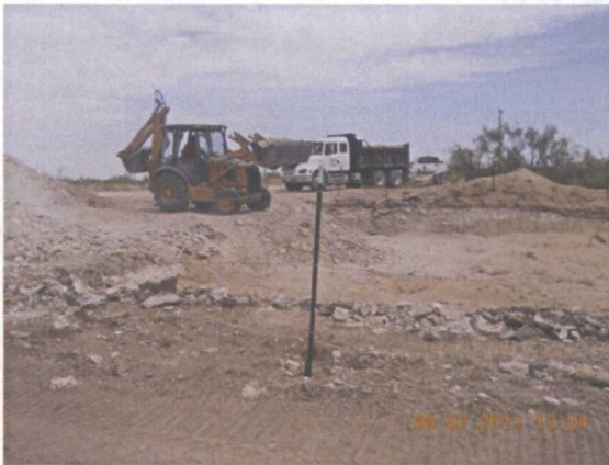
Backfilling over padded liner, facing east 9/8/11
