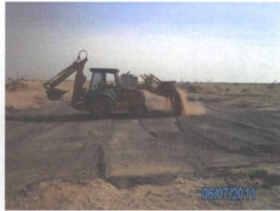
Contouring the backfilled site with imported soil, facing north 6/7/2011
