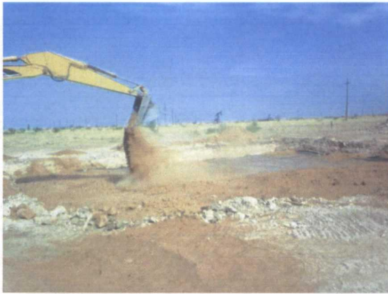
Padding above the liner with 6" of blow sand, facing northwest 6/1/2011
