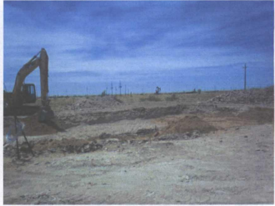
Padding the base of the excavation with 6" of blow sand, facing west 5/27/2011
