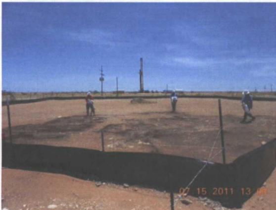
Spreading RestoreNhance on the backfilled site, facing southeast 7/15/2011
