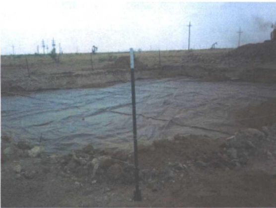
64x63 ft, 20-mil reinforced liner installed at 4.5 ft bgs, facing west 5/31/2011
