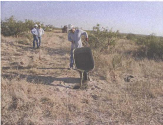
Plugging MW-2 with a 1-3% bentonite slurry, facing north 9/2/11
