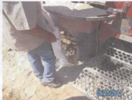
plugging SB-2 with bentonite, facing west
