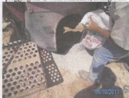
plugging SB-3 with bentonite, facing north
