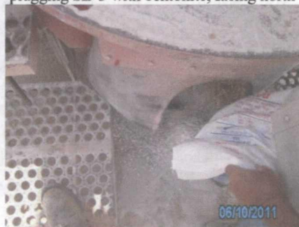
plugging SB-4 with bentonite, facing south
