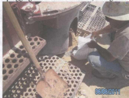
plugging SB-3 with bentonite, facing east
