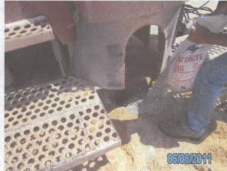
plugging SB-2 with bentonite, facing east
