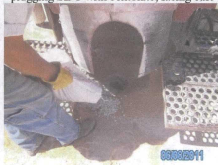
plugging SB-4 with bentonite, facing north
