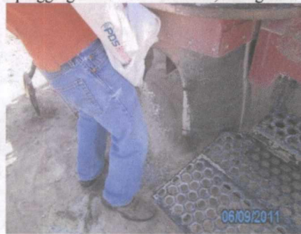
plugging SB-6 with bentonite, facing south
