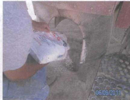
plugging SB-5 with bentonite, facing east
