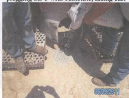
plugging SB-4 with bentonite, facing east
