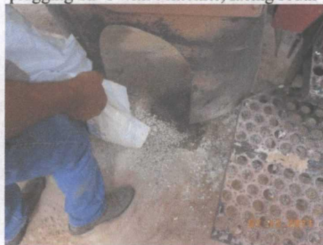
plugging SB-9 with bentonite, facing east
