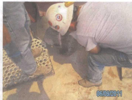
plugging SB-5 with bentonite, facing east
