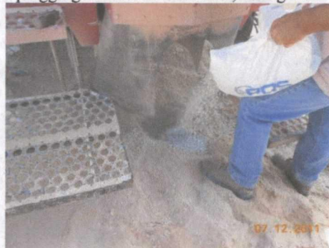
plugging SB-7 with bentonite, facing east
