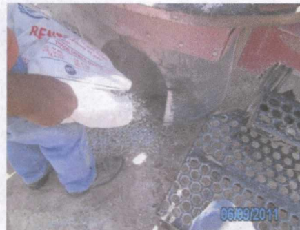
plugging SB-2 with bentonite, facing east
