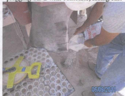
plugging SB-3 with bentonite, facing east
