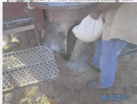
plugging SB-6 with bentonite, facing east
