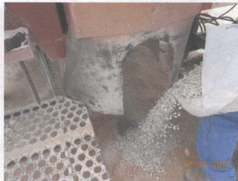
plugging SB-8 with bentonite, facing south
