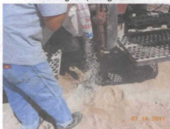
plugging SB-6 with bentonite, facing east
