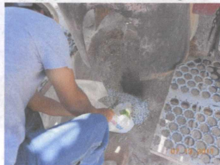
plugging SB-4 with bentonite, facing south
