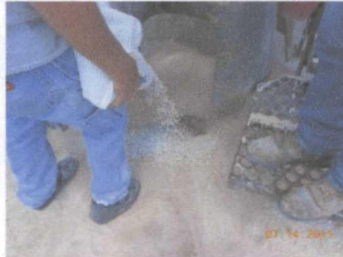
plugging SB-5 with bentonite, facing south
