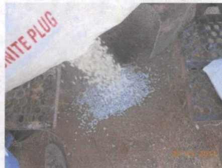
plugging SB-3 with bentonite, facing east
