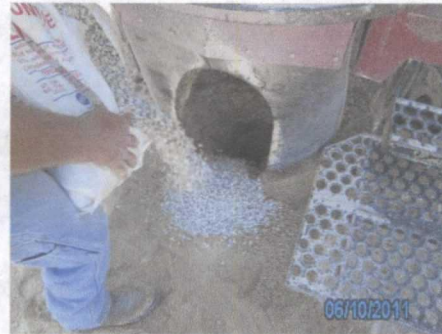
plugging SB-2 with bentonite, facing east
