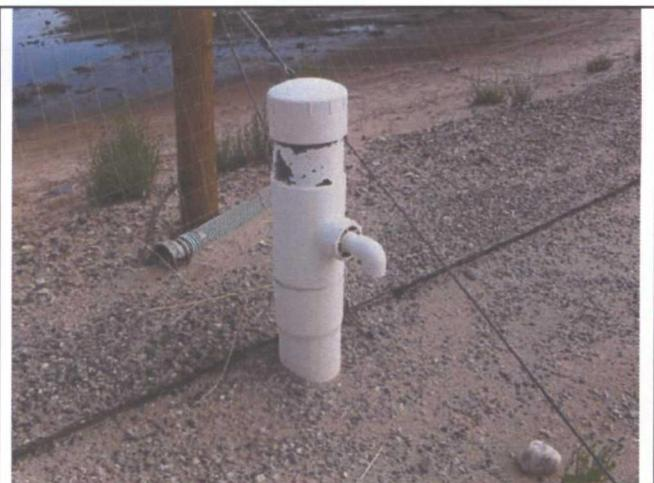
6.) View of leak detection port.
