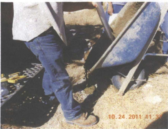
Plugging MW-4 with a 1 – 3% concrete/bentonite slurry
