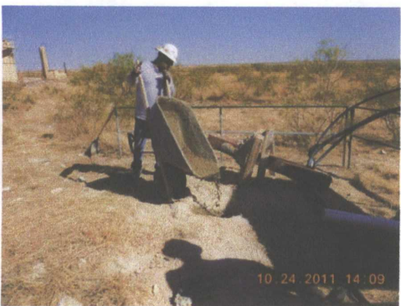
Plugging RW-1 with a 1 – 3% concrete/bentonite slurry
