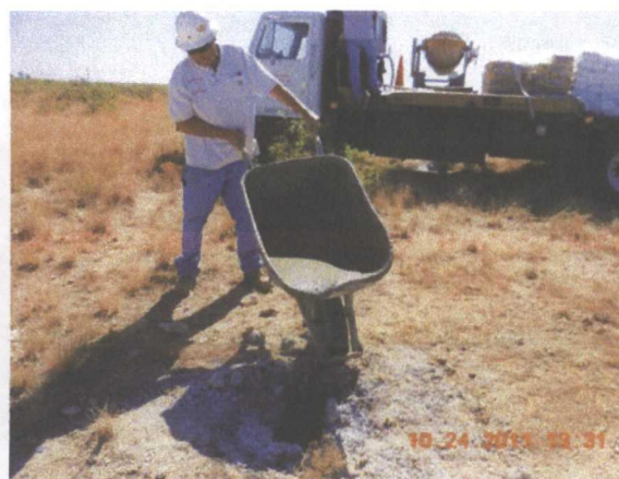
Plugging MW-5 with a 1 – 3% concrete/bentonite slurry
