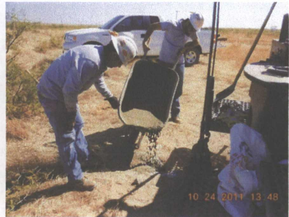
Plugging MW-3 with a 1 – 3% concrete/bentonite slurry
