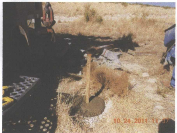
MW-4 plugged, facing west
