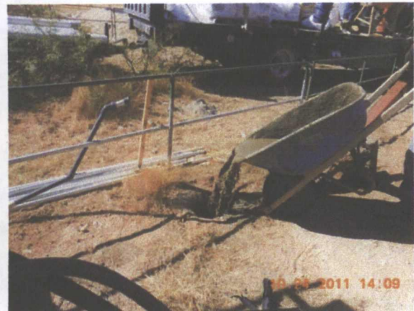
Plugging MW-1 with a 1 – 3% concrete/bentonite slurry
