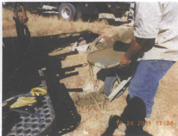
Plugging MW-2 with a 1 – 3% concrete/bentonite slurry
