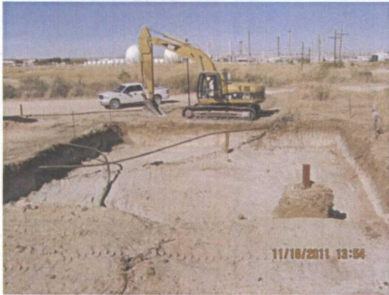
completed 51x44x5-ft excavation, facing north 11/18/2011
