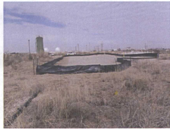
site complete with silt net fencing, facing south 12/15/2011
