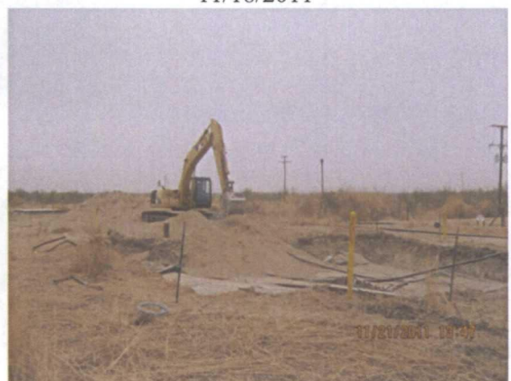
backfilling site with blended soil, facing south 11/22/2011
