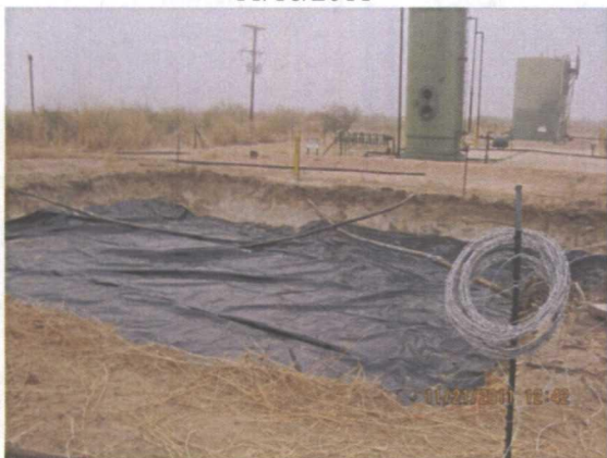
51x44-ft 20-mil, reinforced liner installed, facing west 11/21/2011
