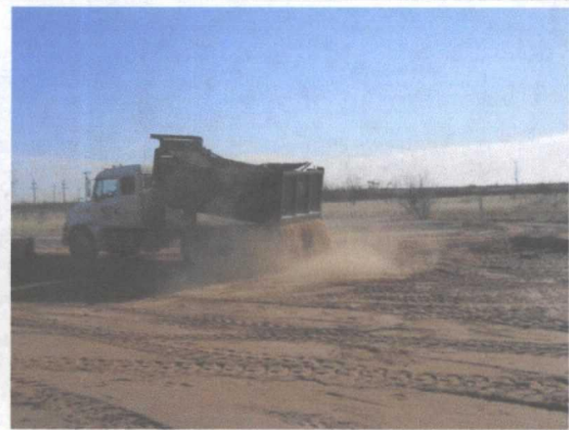
importing clean soil to contour the site, facing east
