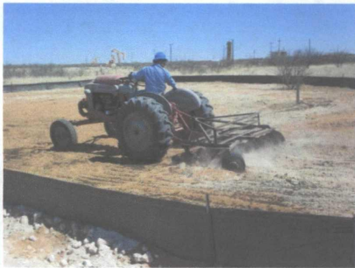
tilling in seed and bioNhance, facing northeast
