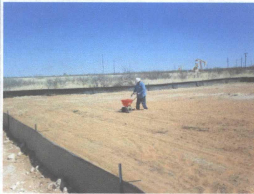
seeding the backfilled site, facing north
