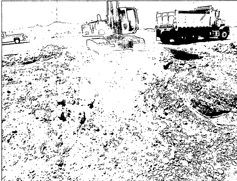
Photo 7: View of excavation to approximately 7 feet bgs in heavily impacted area (looking west).
