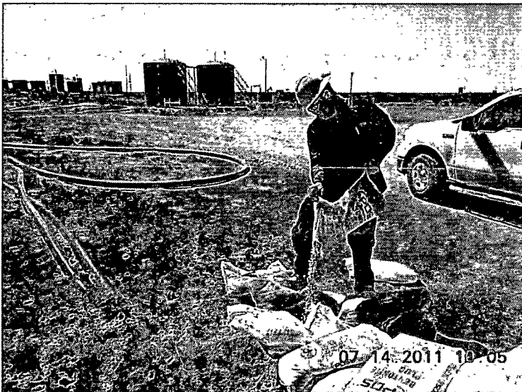
Plugging MW with bentonite, facing SE 7/14/2011
