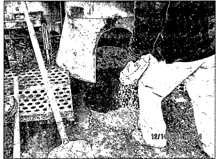
Plugging SB1 in total with bentonite
