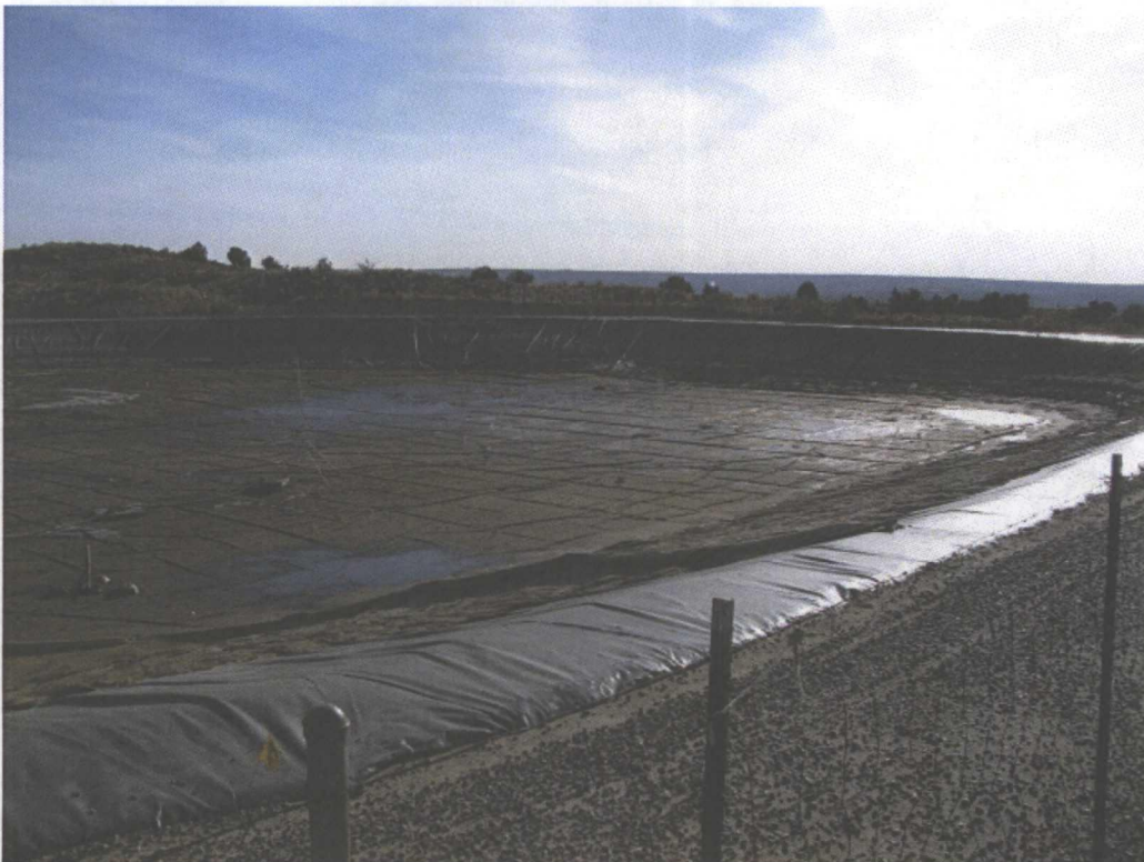
Photograph 2: Western portion of the waste water evaporation pond after removal of fluids and a majority of the sludge/sediment. Pond liner still in place. Facing Southwest.
