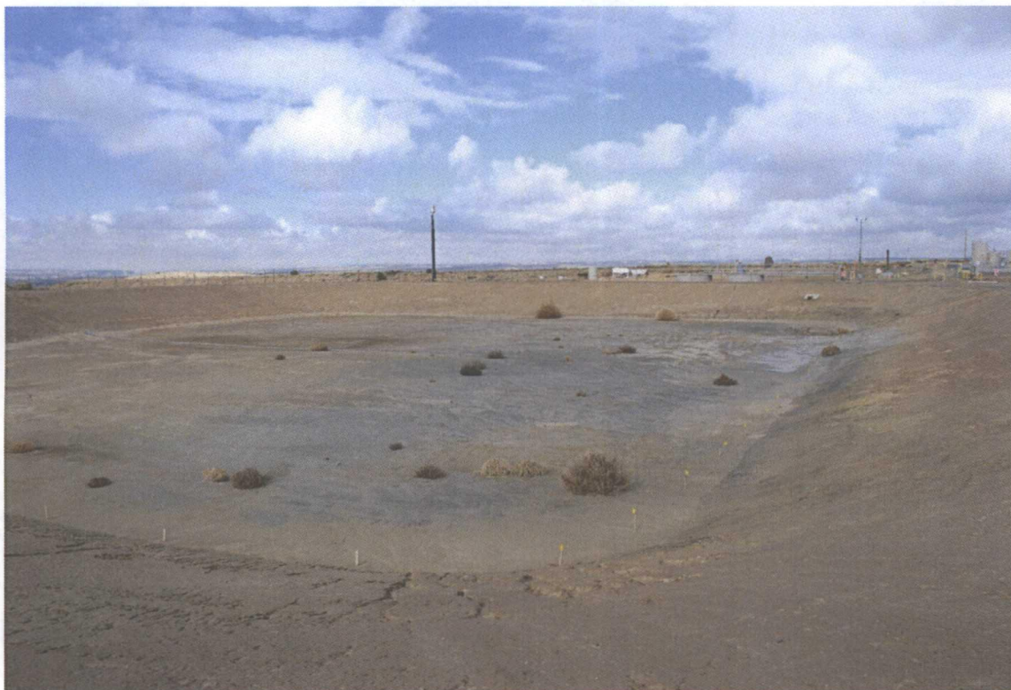
Photograph 3: Eastern portion of the waste water evaporation pond after removal of pond liner. Facing North.
