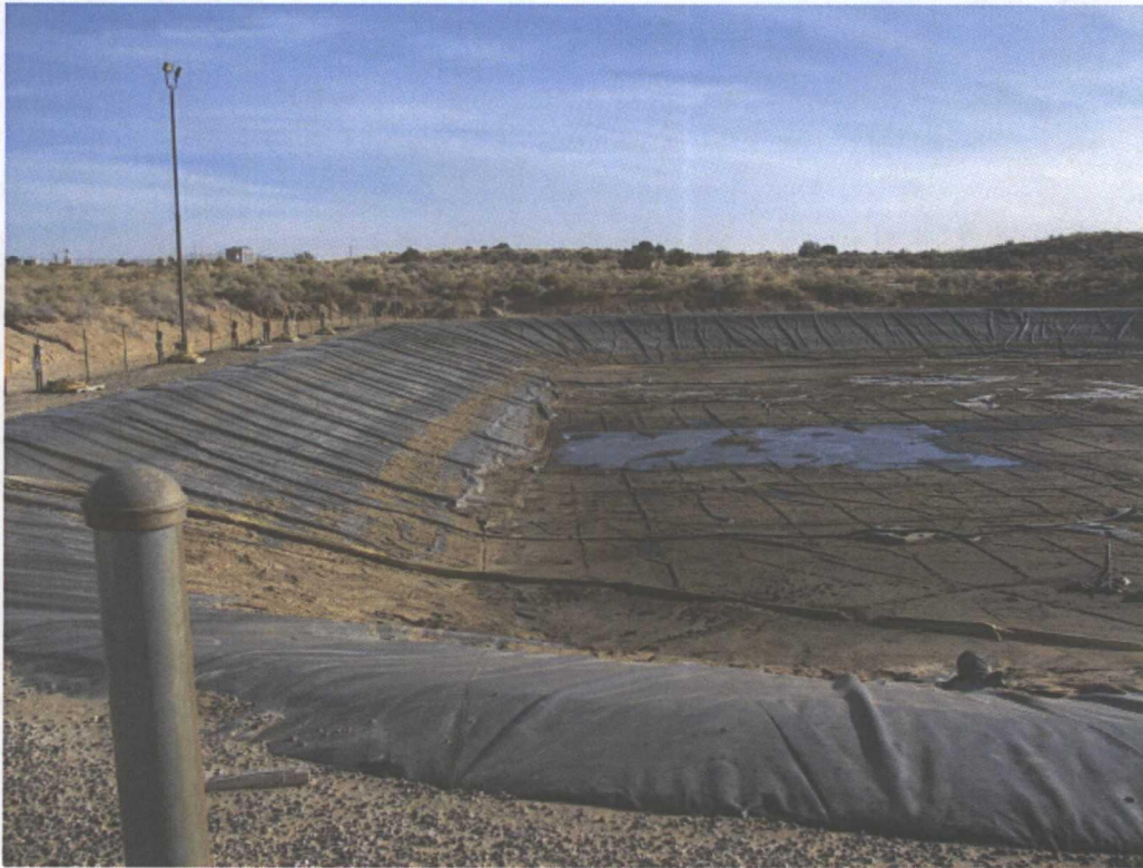
Photograph 1: Eastern portion of the waste water evaporation pond after removal of fluids and a majority of the sludge/sediment. Pond liner still in place. Facing South.
