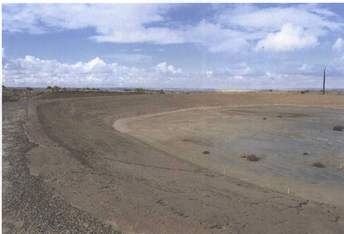
Photograph 4: Western portion of the waste water evaporation pond after removal of pond liner. Facing Northwest.
