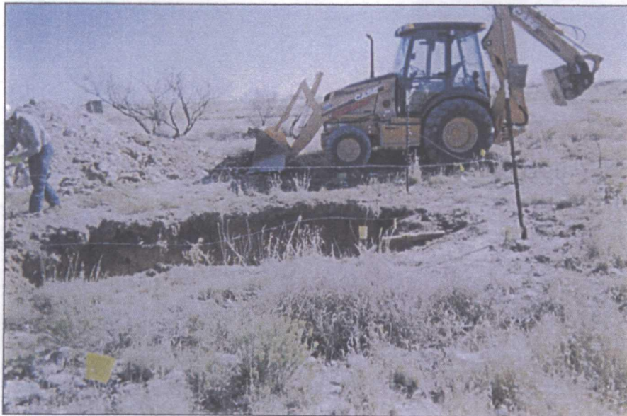
backfilling trench
