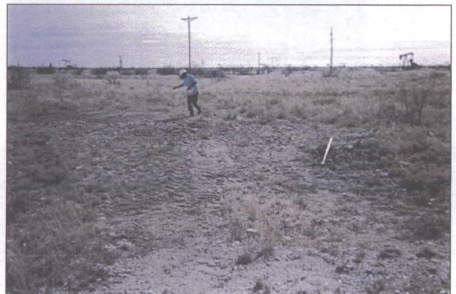
seeding disturbed surface after backfill 11/23/2005
