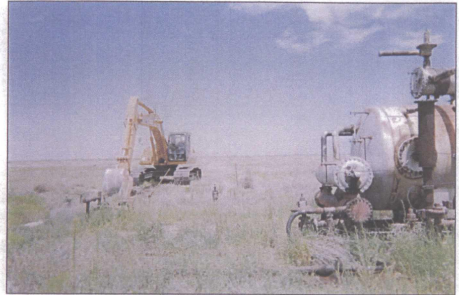
delineation trench at former junction box site
