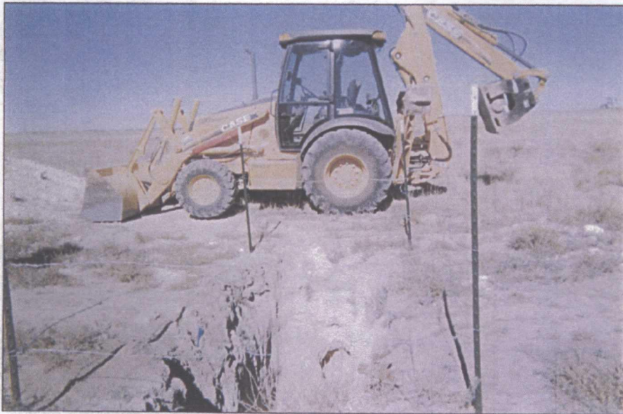
backfilling delineation trench
