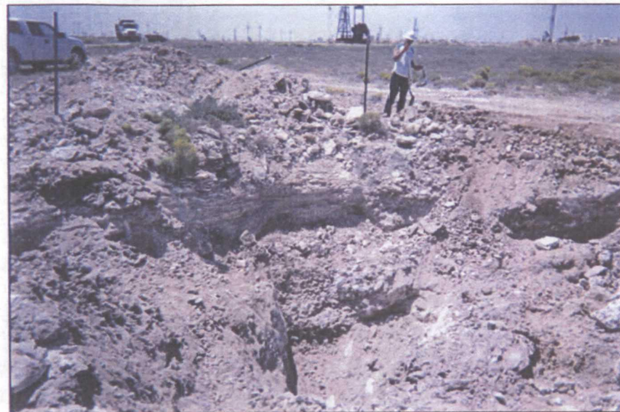
9-ft delineation trench prior to backfill
