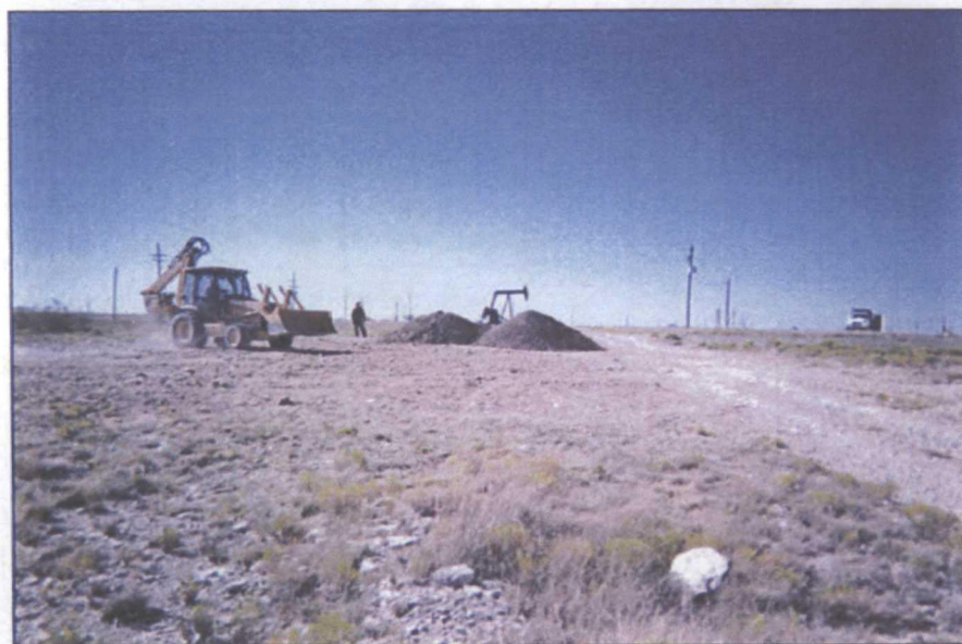
spreading imported soil
