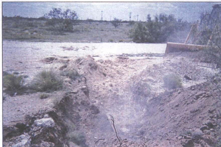
backfilling trench
