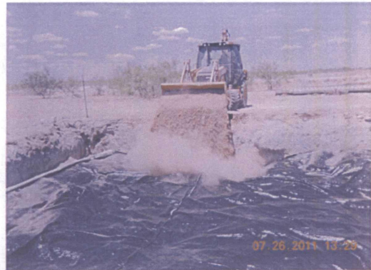
Backfilling site with imported soil, facing north 7.26.11
