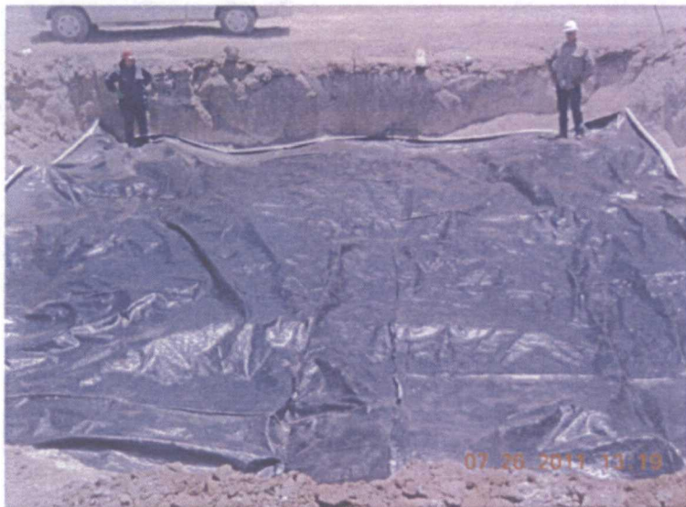
Installing 30 x 30 20-mil reinforced liner at 5-ft. BGS, facing south 7.26.11
