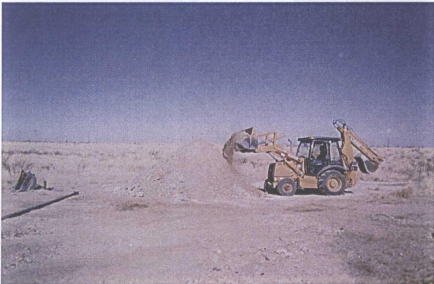
Blending backfill
