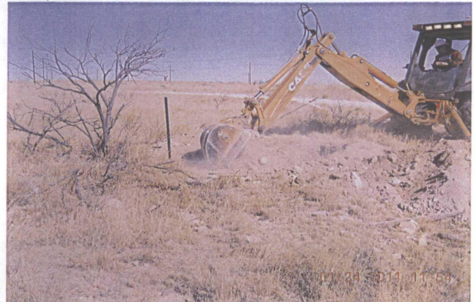
Backfilling with clean imported soil, facing north
